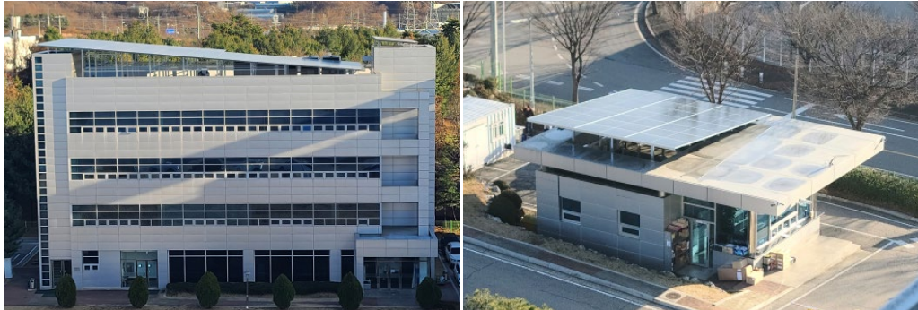
Solar Power Facility Installation at Hwaseong Plant: Left - Welfare Building Roof, Right - Security Office Roof
